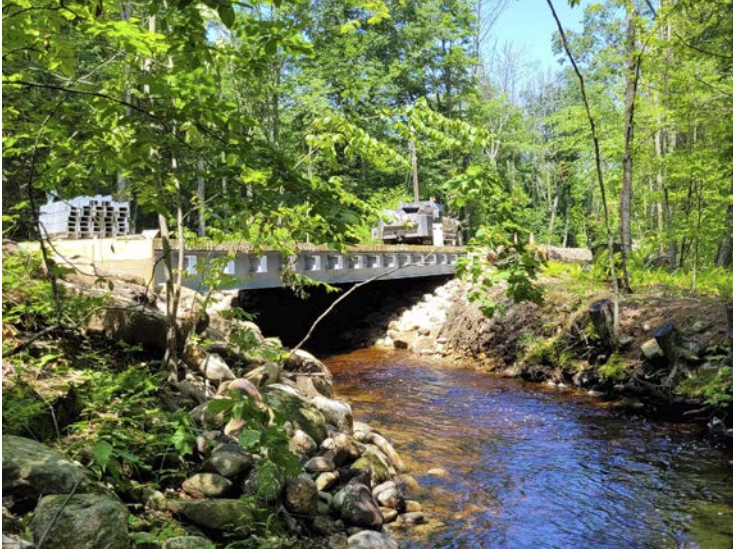
Brook Rd. Bridge Project 2023
