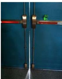
Figure 7 - Exit doors with no weatherstripping
