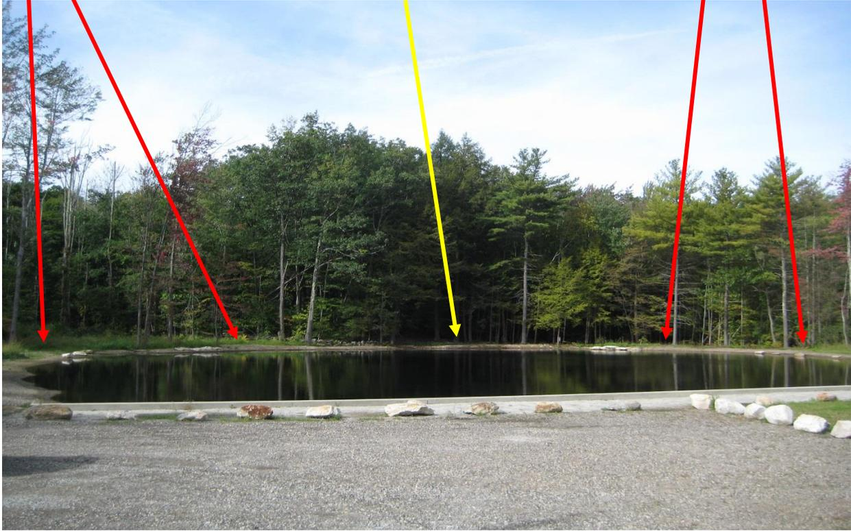
Right hand side path still needs to be raise to assist with walking surface and controlling water from swamp from flowing directly into the pond
